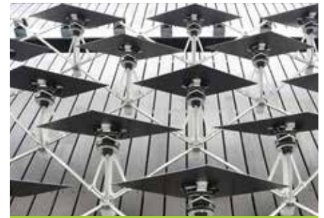
Image 2 - Adaptive solar façade - Second implementation of ASF prototype at the NEST site in Dübendorf, 2017
