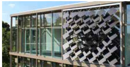
Image 1 - Adaptive solar façade - First implementation of ASF, HoNR at ETH Zurich, 2015
