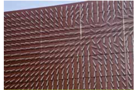
Image 6 - A wind-driven kinetic façade on the blank wall of the Randal Museum in San Francisco, by Charles Sowers Studios
