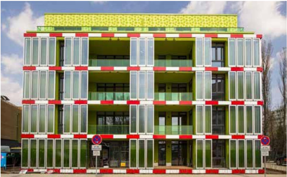
Image 3 - Algae-Based Bioenergy Façades at the Bio Intelligent Quotient (BIQ) building in Hamburg, Germany
